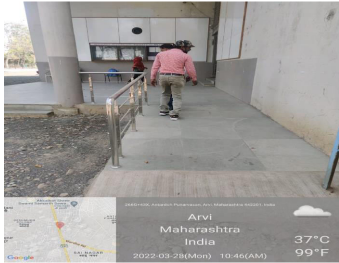
Ramp (Disabled friendly facility)
